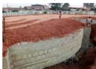
Construction work as at December 7, 2020
