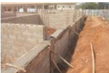
Construction work as at November 2020
