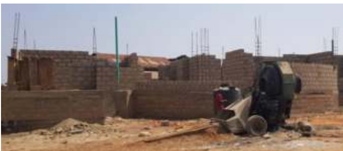
Construction work as at December 26, 2020
